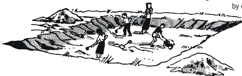
**Dugout Ponds** are built in flat areas by digging out the soil. Water level is below the original ground level.
