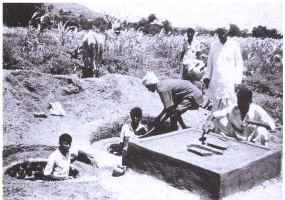
Building a twin pit pour-flush (water-seal) latrine. (Photo: Philip Wan, UNICEF)
