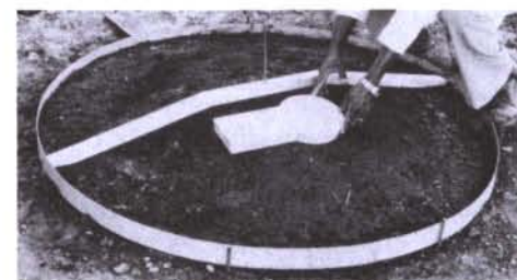
Preparing to make an un-reinforced domed concrete slab. (Photo: R Franceys)
