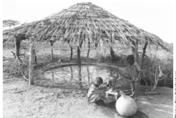
Children using a small hand pump in front of a small water tank covered to slow evaporation and keep out livestock and children.
