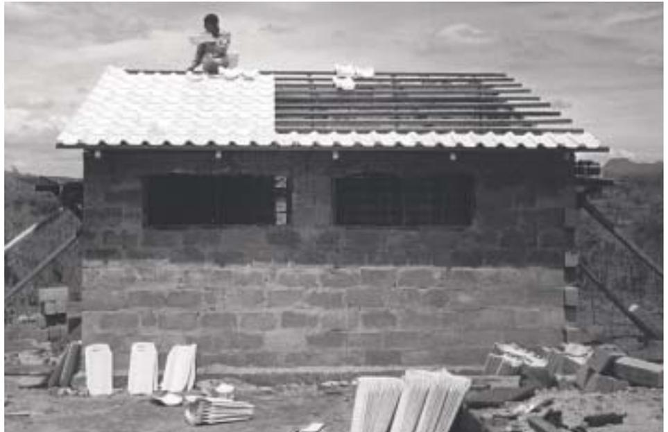
*A tiled roof needs a strong roof structure. Tiles are heavier than metal sheets. The roof will need to be well constructed with accurate measurements and level cross beams.*
