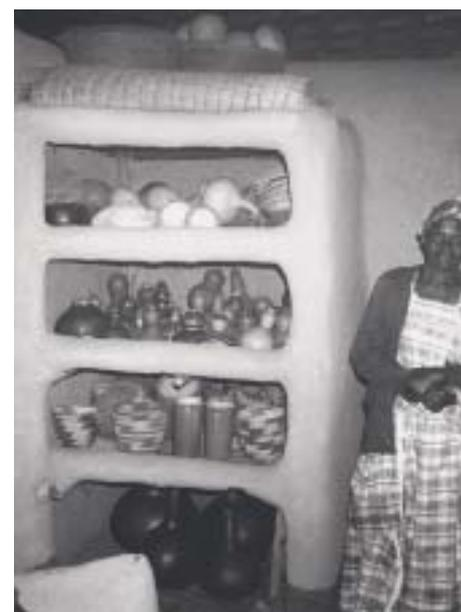
The photo shows the proud owner of an impressive-looking kitchen cupboard in Rukungiri, Uganda. Mud and cement plaster coats a wooden framework. The mat on top can be rolled down to close the cupboard.
