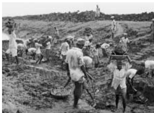
Digging the canal.
