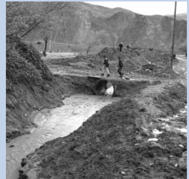
Shibanai village, Tajikistan, after 24 hours of heavy rain. The drainage canal has silted up. When it rains, blockages increase the danger of burst banks and flash floods. Water is slowly seeping up the walls of the houses. Mosquitoes are attracted to the stagnant puddles. Oxfam has paid for a mechanical digger to clear the canal.
