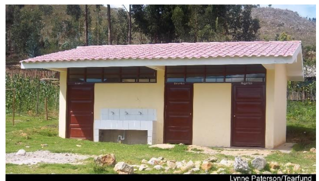
Photo: Segregated latrine block in Peru with water source
