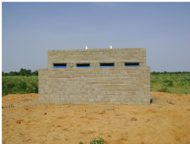
Fig 1. Latrine constructed with SSBs
